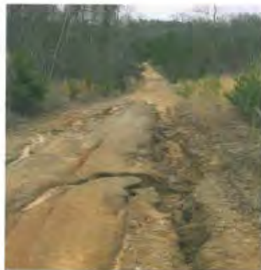
Abandoned Dirt Pits, Abandoned Surface Mines, and Access Roads that Need Stabilization
