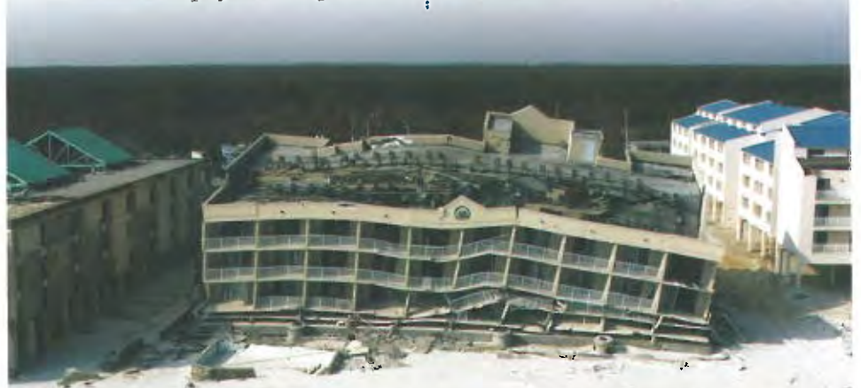
Damage to beach front condos in Gulf Shores, Alabama from Hurricane Ivan.
